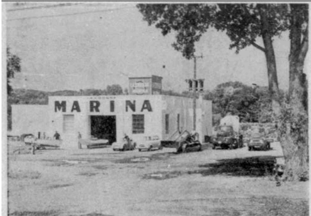
NEW MARINA —This is the site of La Crosse Marina, Inc. The marina is on the West Channel and its vehicle entrance is across from Pettibone Park. Crews are working to get the marina in full operation soon and when finished it will provide dockage for 400 boats.—Tribune Photo.
